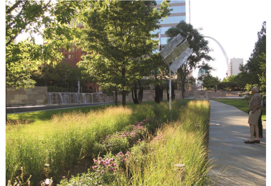
Six rain gardens cover over 5,000 square feet of area that collect and infiltrate stormwater from over two-thirds of the site. Rain gardens are planted with native grasses and wildflowers - in this case, with Switchgrass ( Panicum ) and Bee Balm ( Monarda ).
