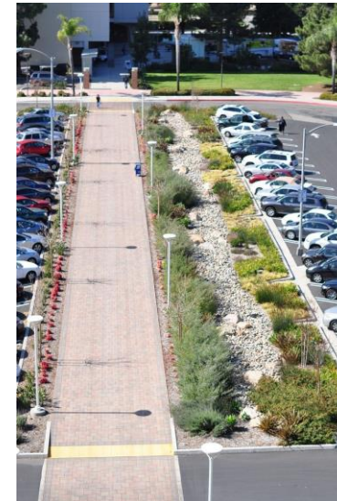
Six rain gardens cover over 5,000 square feet of area that collect and infiltrate stormwater from over two-thirds of the site. Rain gardens are planted with native grasses and wildflowers - in this case, with Switchgrass ( Panicum ) and Bee Balm ( Monarda ).
